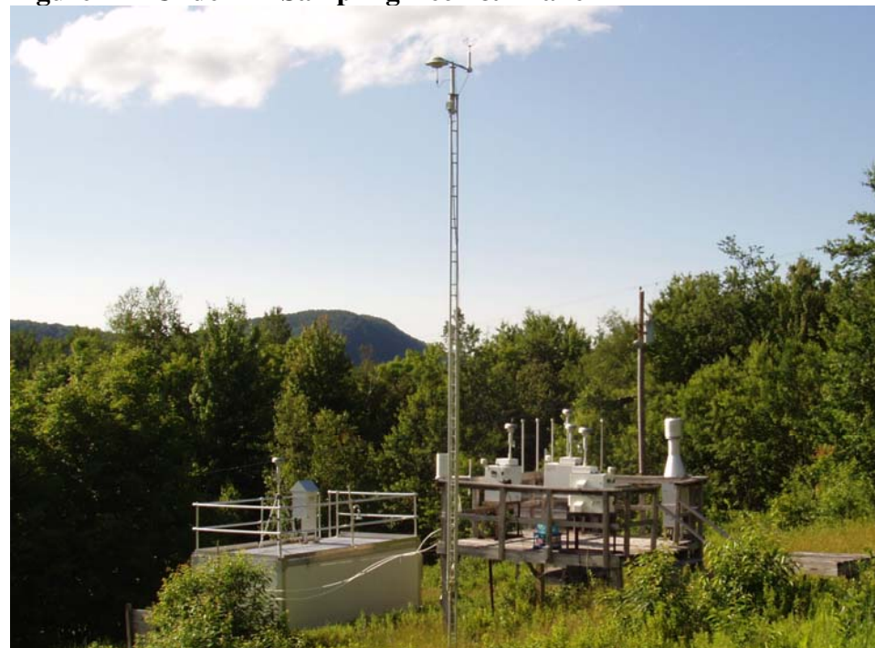
Figure 11 - Underhill Sampling Deck & Trailer
