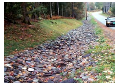
A stabilized road ditch.
