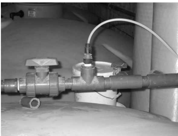
Figure B - This is the proper way to install the Chlorine Injector Check Valve Assembly (note that injector Tee should be Brass or PVC to resist corrosion)
