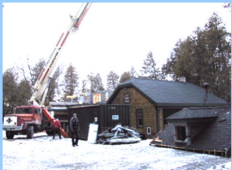
A "deconstructed" home in Charlotte. Deconstruction saved $3,400.
