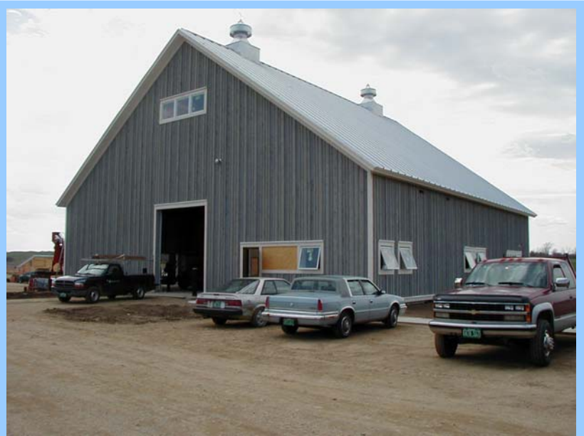
Newly constructed Material Recycling Facility at Middlebury College.
