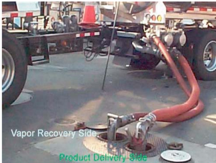
Stage I Gasoline Vapor Recovery using Dual (Two-point) System
