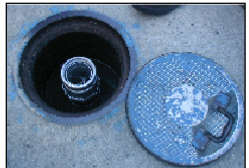
Sample Spill Protection
